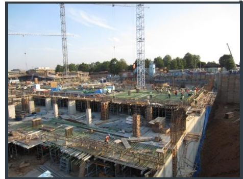
Figure 7: Concrete Slab Construction
