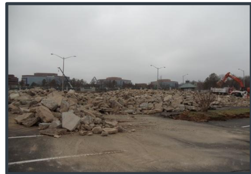
Figure 5: Demolition of Parking
