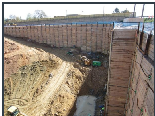
Figure 8: Soldier Piles and Lagging
