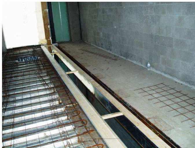
Figure 13 - Expansion Joint Section Photo Courtesy Jim Boje, PE (Wendel)
