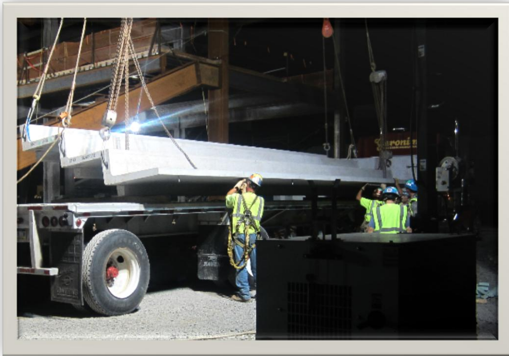
Photo 1: Precast Stadia | Courtesy of Mortenson
