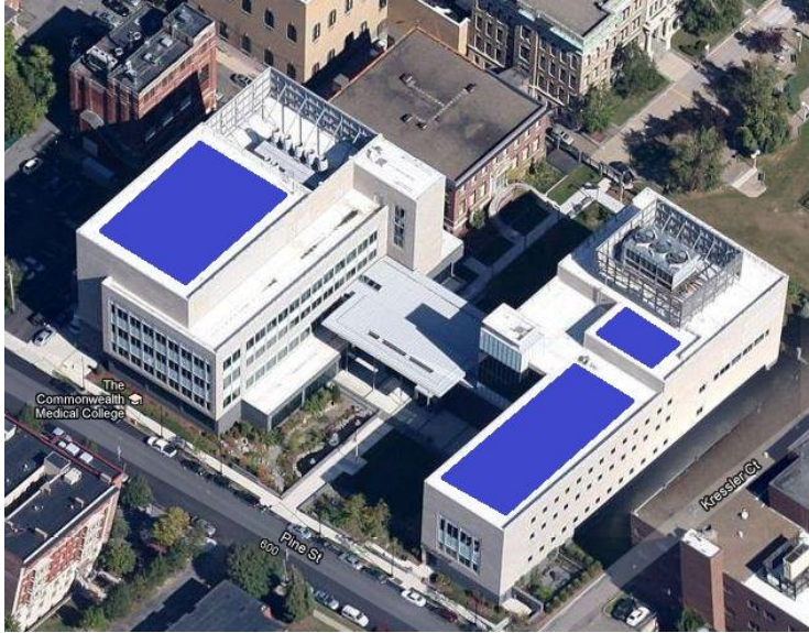
Figure 70.1, Area in blue is where the solar panels were placed. Image from google maps, edited by the author
