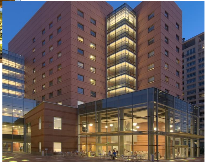
Figure 62, Top, Taken directly from Boston Valley Terra Cotta's website, is The Bechtler Museum of Modern Arts. The rainscreen cladding here are the same size of a normal brick. This shows that many sizes are possible when using TerraClad Rain Screen. This building also shows the color of stones similar to ones that are used in TCMC. The size and color can keep the architectural look similar to the original.
