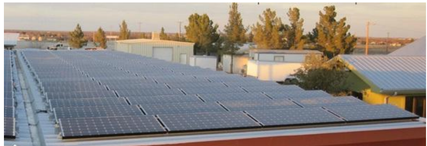
Figure 70.2, Image of installed HIT 220A solar panels. This is how TCMC roof, where solar panels were placed, will look. Image from Panasonic Sanyo HIT Technology
