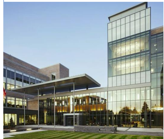
Figure 2 Picture of the exterior showing the glass and brick facade on the TCMC. The Tower is shown, made will all glass walls. http://www.hok.com
