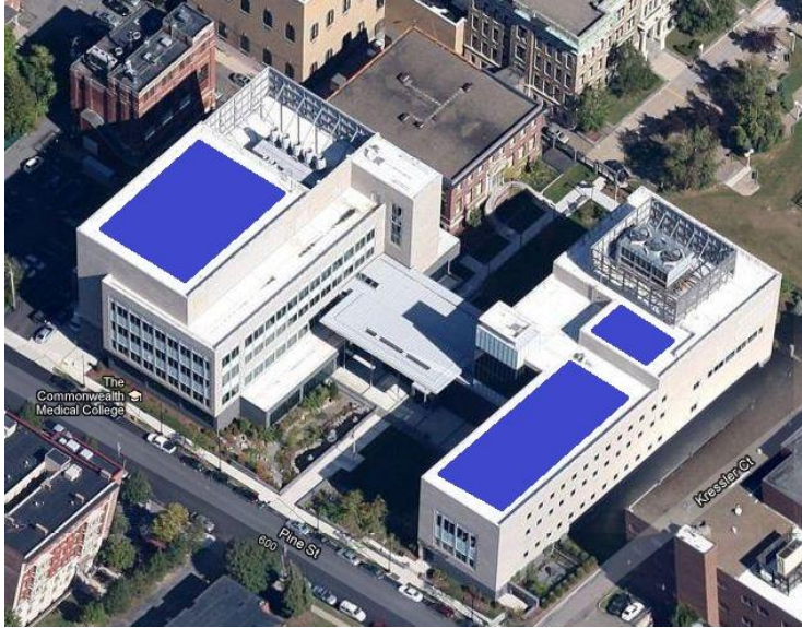
Figure 70.1, Area in blue is where the solar panels were placed. Image from google maps, edited by the author
