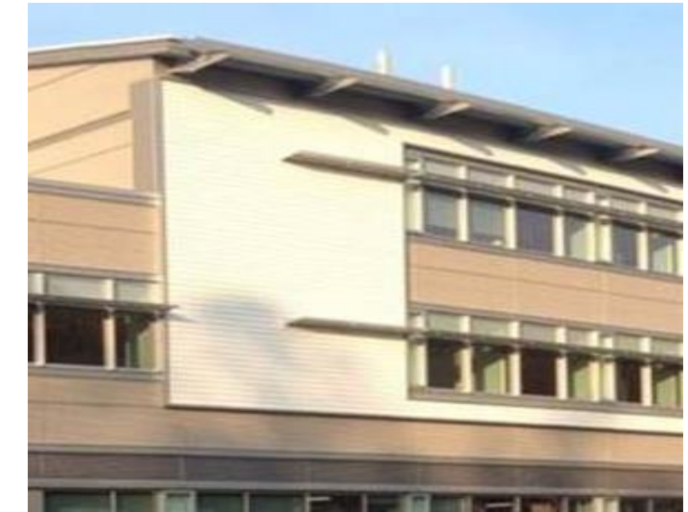
Fiber Cement Siding
