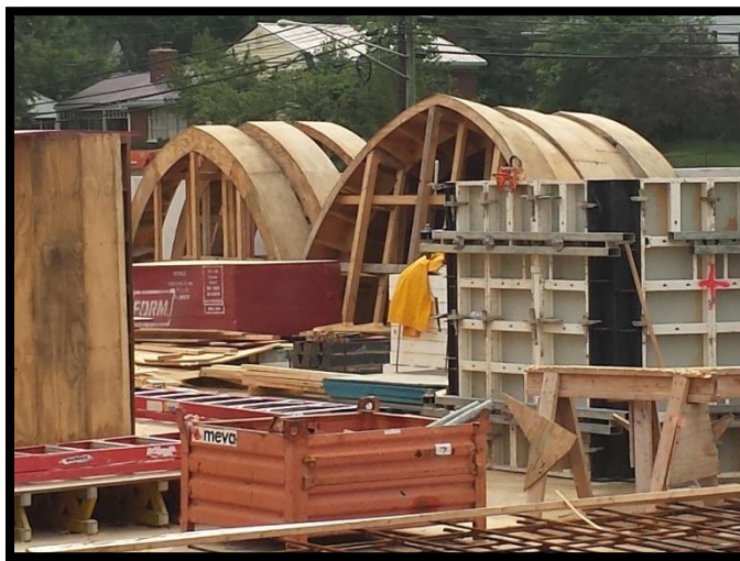
Figure 8 Custom Arch Formwork
