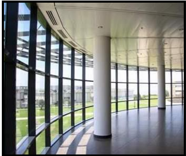
Butt Glazed Curtain Wall
