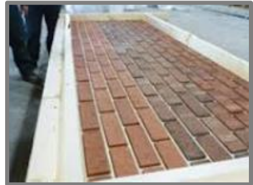
Figure 4.1: Proposed prefabricated precast brick veneer.
