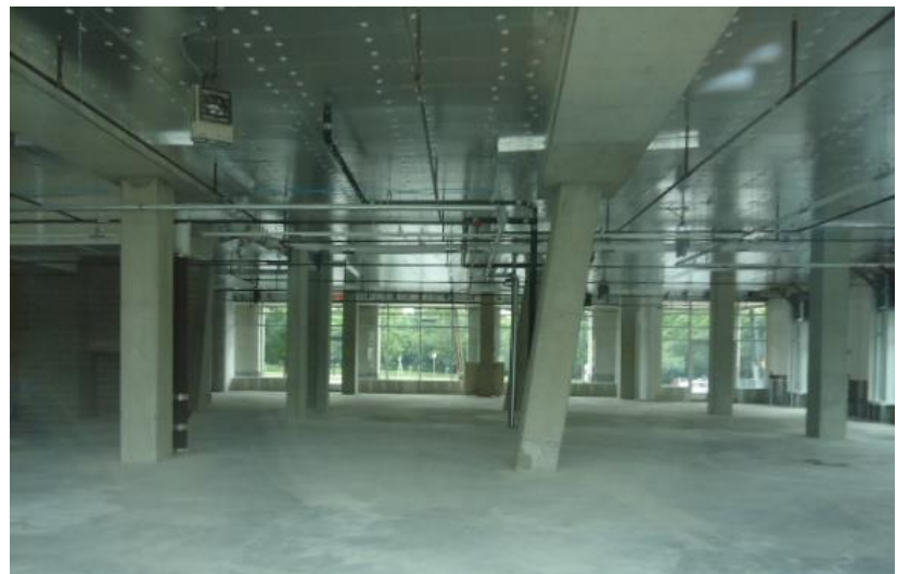
Figure 8: Sloped Columns in Retail Space
