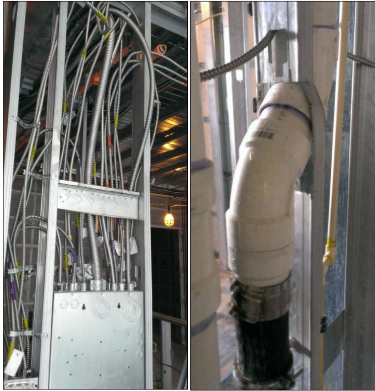
Figure 12: Examples of MEP Construction with Infinity
