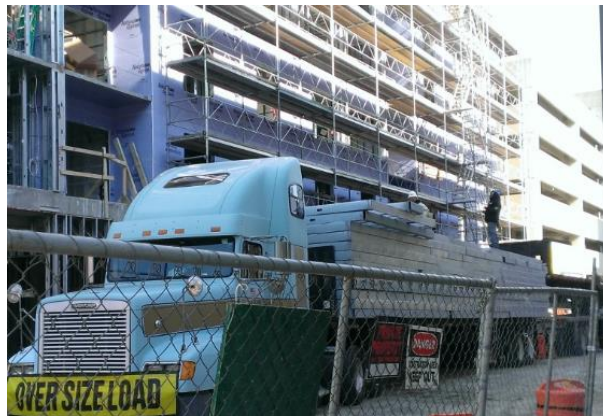
Figure 9: Flatbed delivering Infinity Panels on site.
