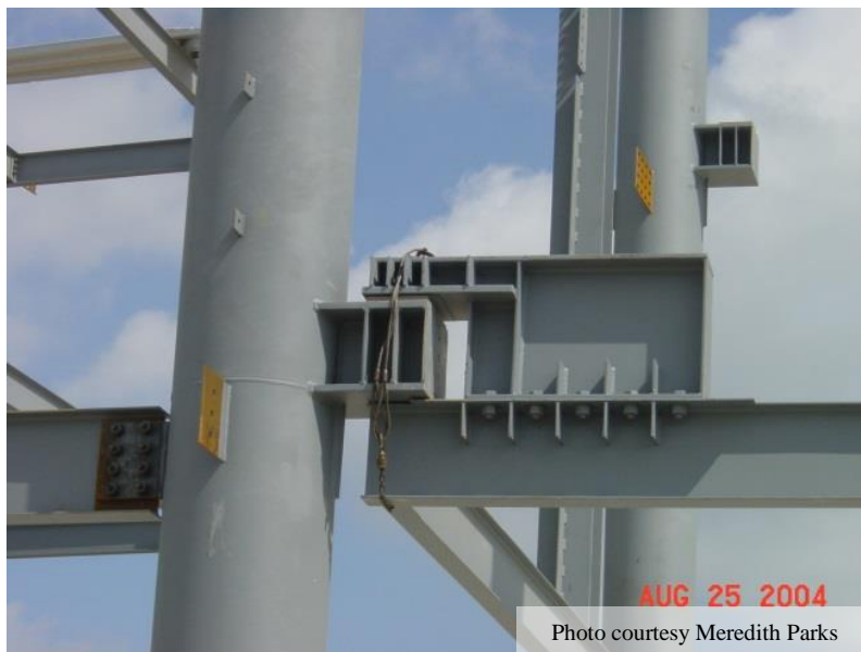
Figure 14: Photograph of seismic joint
