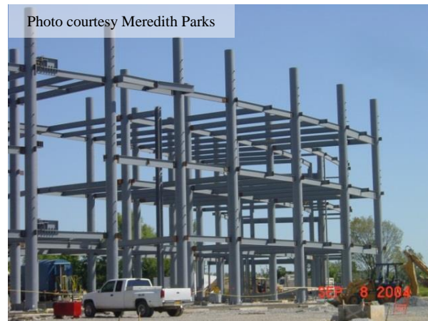
Figure 6: Photograph during erection of HSS framing
