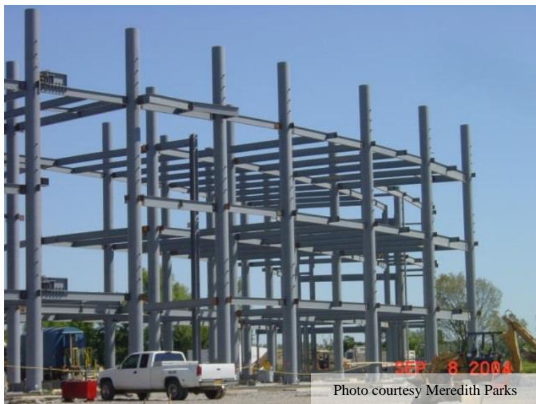
Figure 67: Construction photo with no evident LFRS
