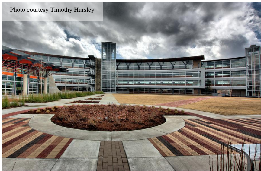
Figure 98: Exterior shot of natural daylighting penetrating building façade
