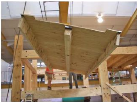
Figure 108: Semi-prefabricated TCC floor system in New Zealand (Yeoh et al.)
