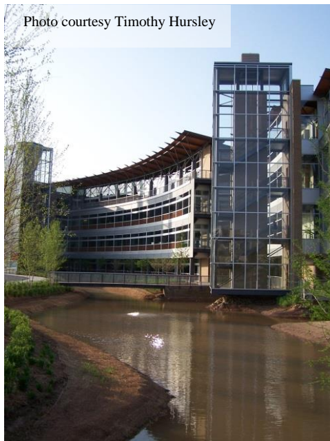
Figure 95: Water collection system tower (far left) and local wetland (front right)
