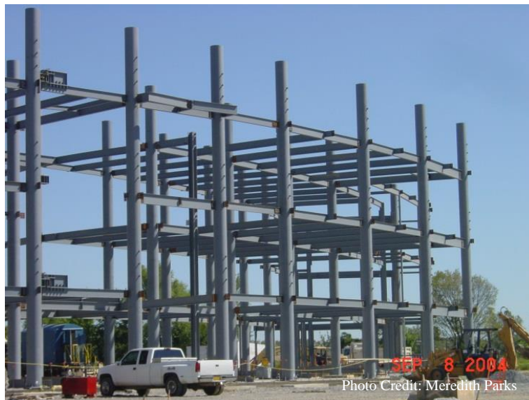
Figure 11 | Photograph during erection of HSS framing
