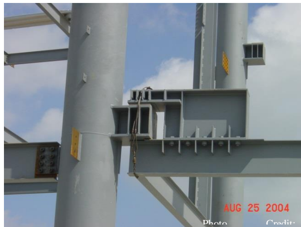
Figure 19 | Seismic Joint, detail (above) and photograph (below) (Drawing 3/S500), allows for natural movement of the building
