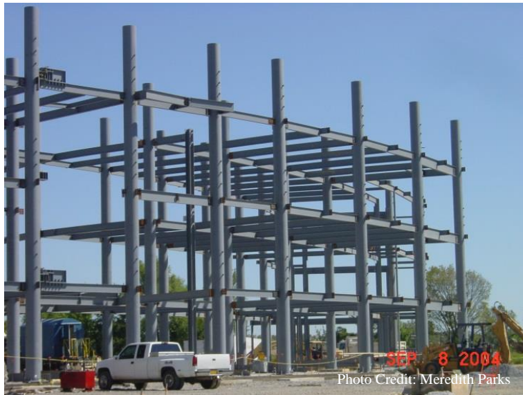
Figure 11 | Photograph during erection of HSS framing
