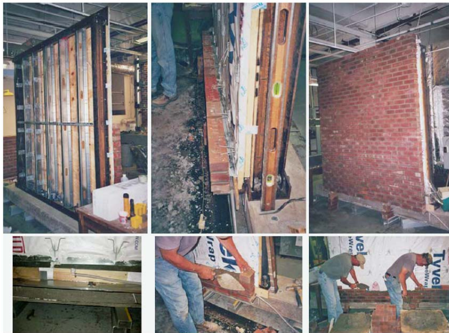
Figure 23: PBVSS mock-up during construction (Liang and Memari 2011)
