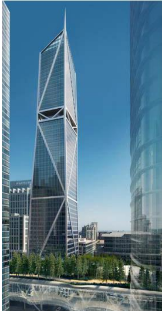
Figure 1 | Southwest Elevation View (Courtesy of Heller Manus)
