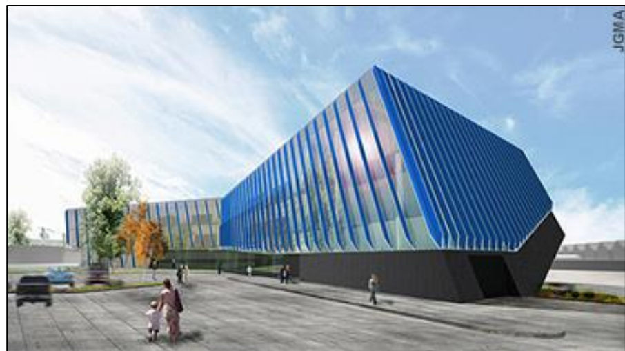
Figure 4 – El Centro’s solar fins were designed to limit solar gains into the building
