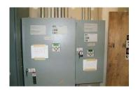
Two main panels draw from the local utility, one at 4000A 480Y/277V 3ø the other at 3000A 480Y/277 3ø. The first panel is dedicated to the main hospital building, which includes the Woman's Pavilion. The second serves the central energy plant building and off its equipment including the cooling towers. The main hospital panel serves 10 separate panels without stepping down in voltage. From those 10 distribution
