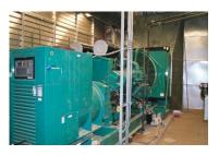
power from a 1250kW/1562kVA Diesel Generator to keep life support systems functioning at all times. Multiple surge suppression devices are located on each major panel to ensure safety of the system from overload.
