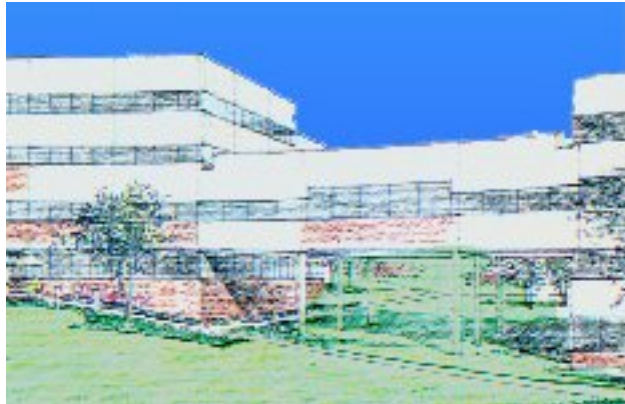
Figure I-1 Artist rendering of the sky bridge between The Medical Office Building (left) and its neighbor
