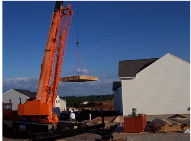
Figure 7: Panel being picked with a crane.
