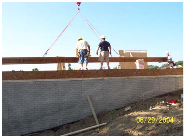
Figure 9: A first floor panel being installed.
