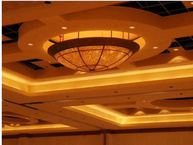
Figure 10: One Type of Existing Incandescent Ballroom Fixtures
