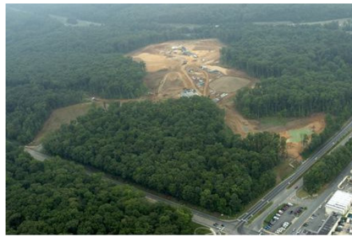
Figure 6 – Construction Site Conditions
