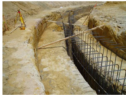
Figure 1 – Shear Key Footing System
