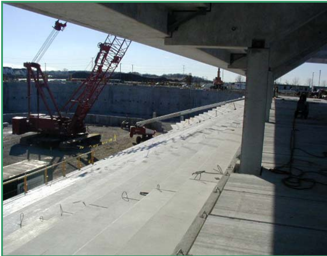
Interior Bowl Construction
