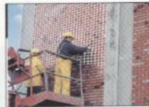
After the panels are tilted and erected, the snap carriers are removed.
