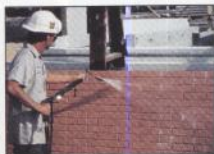
Panel is cleaned to remove concrete leakage.
