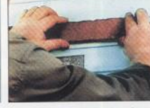
Latex modified mortar bonds to the bricks and clips, creating a permanent mechanical connection to the structure.
