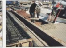
Concrete is placed and vibrated on panels.
