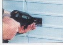
Panels are installed with interlocking clips that mechanically lock the panels and bricks to the structure.
