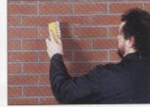
Brush joints to remove excess mortar before mortar cures.
