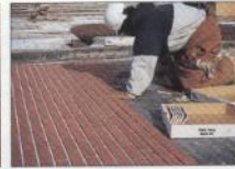
Assembly of Brick Snaps for Tilt-Up is fast at the rate of 2 to 3 square feet per minute, per man.
