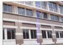
Precast thin brick panels eliminate the need for lintels, sills, weep holes and tie rods.
