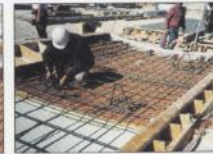
Re-bar and clips or anchors are assembled before concrete is placed.
