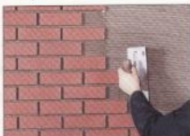
Mortar is applied with a 1/4" notched trowel.
