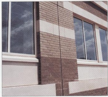
Two of the three colors are shown in this panel area with custom size brick (2 1/8" x 1 1/8" x 1/4") produced for this building.
