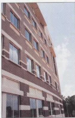
Three custom colors were installed as shown on this curved wall.
