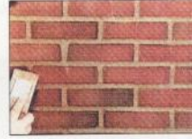
Installation is cleaned with a brush to remove excess mortar.
