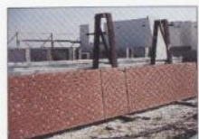
Brick precast panel ready to be cleaned.
