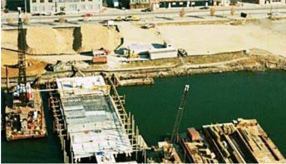
Picture A: Floor plank assembly
