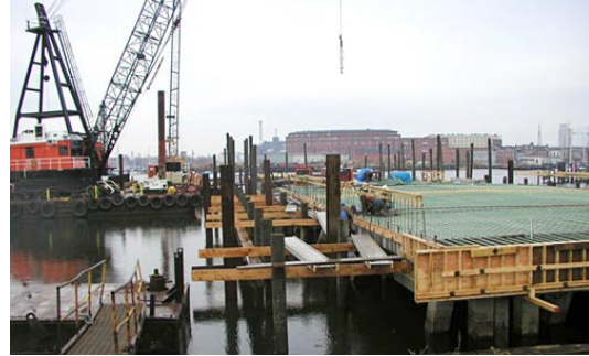
Picture B: Parking/Pier level
