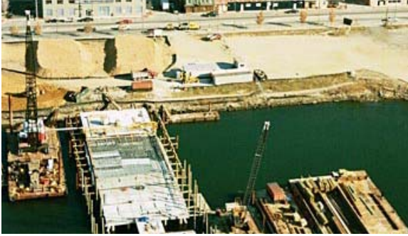
Picture A: Floor plank assembly
