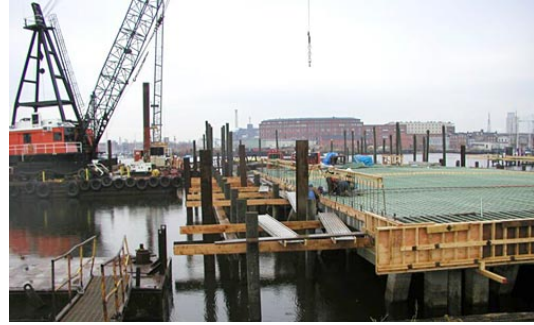
Picture B: Parking/Pier level
