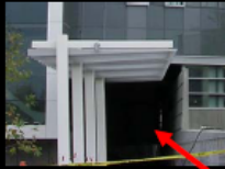
Downlighting on open canopy for entrance to tunnel
