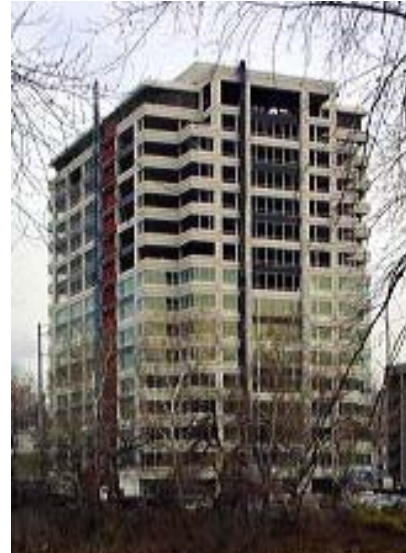
Figure 4: Construction of Eight Tower Bridge
