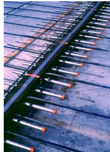
Figure 9: Post tensioned slab www.utexas.edu
