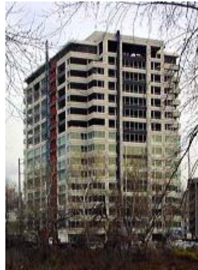
Figure 4: Construction of Eight Tower Bridge
