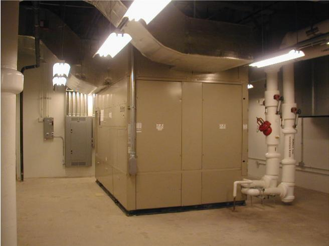
Figure 2.3A. McQuay Packaged SWP Air Handling Unit in Third Floor South Mechanical Room.
