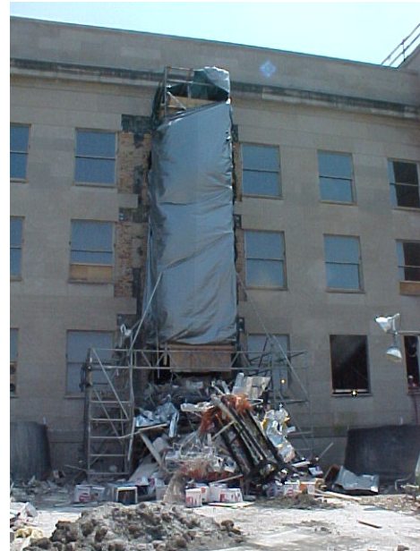
Fig. 2 - Trash chute in demolition area.
