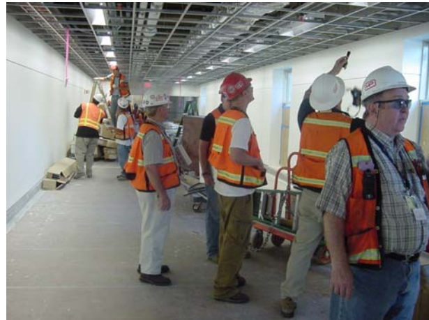
Figure 1 – The quality control team performs a ceiling close-in inspection.
