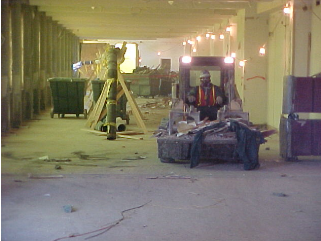
Figure 1 - A bobcat removes trash in Wedge 3 demolition area.
