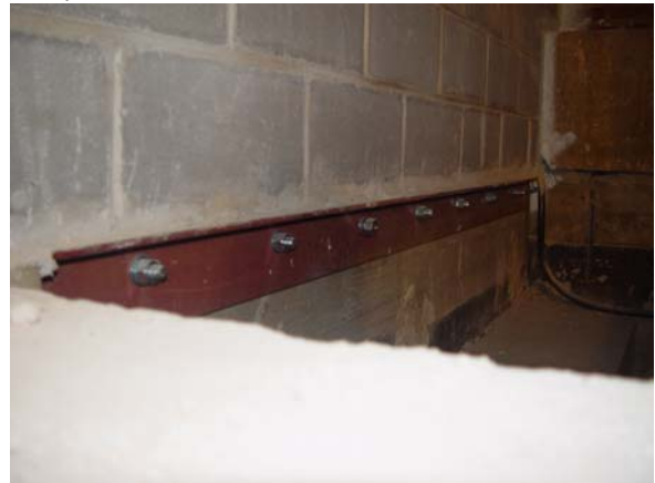
Fig. 2 – Angle reinforcement at a new penetration and CMU wall.
