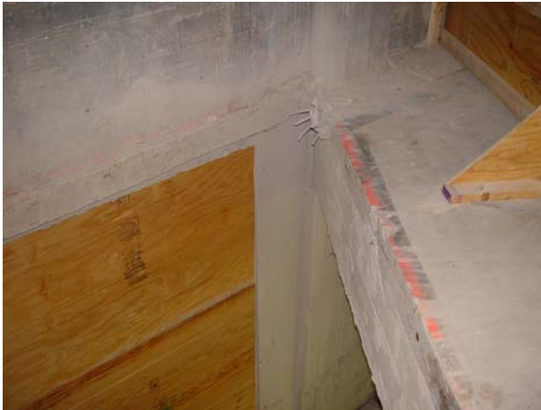
Fig. 1 – A typical new concrete penetration in Wedge 3.
