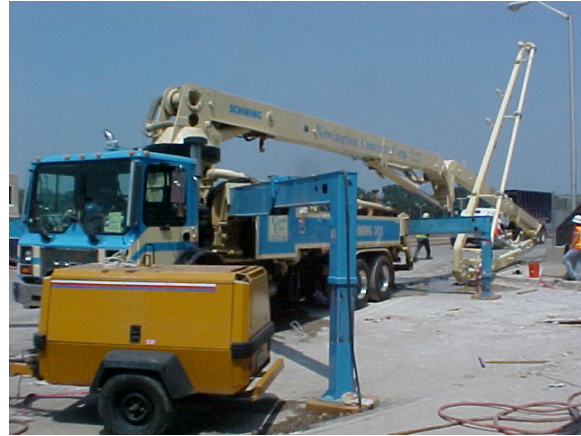
Fig. 2 – Concrete truck and boom pump on site.
