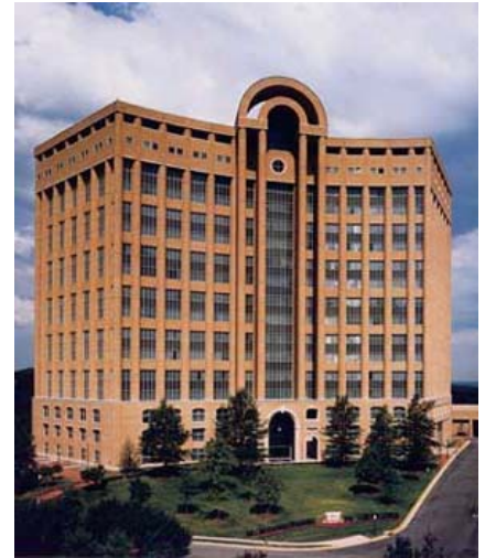
Towers Crescent Building
