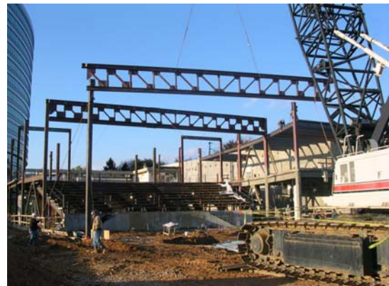
Figure 1. Placement of Steel Trusse
