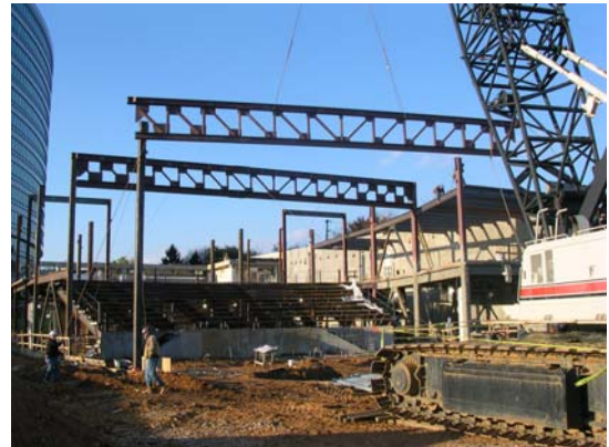
Figure 3. Placement of Steel Trusses
