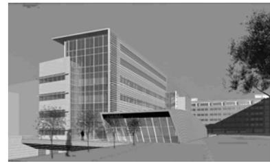
pre-cast panels; however, this system also weighs the same as the current system, 11psf. There would be a slight increase in the structural members, due to the increased area of cladding vs. glazing of the traditional layout as compared to the modern one. The new typical member sizes are W27X84, W24X55, and W21X44.
