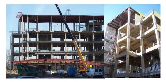
The current system also has steel construction in the penthouse area with the typical steel column being either W14X122 or W10X73. The steel beams in the penthouse roof, as well as the high-bay laboratory are typically a W14X32, W12X21 with secondary beams typically being either a W10X17 or a W8X15.
