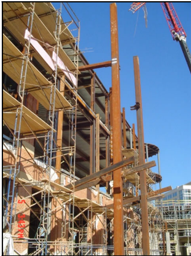
Current Photos of Curtainwall Erection.
