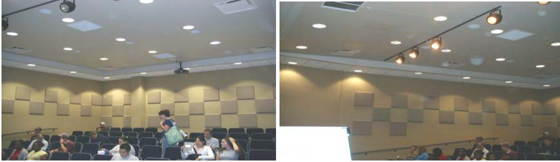
More pictures of the auditorium classroom/ video conferencing room. The picture on the right shows a close up of the track lighting, and the somewhat disturbing difference in CCT between the wall wash + down lights vs. the track lights.
