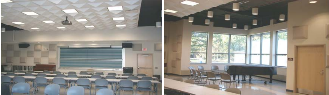
More pictures of the Pechter Family Music Room. The picture on the right shows a closer view of the recessed cylinder luminaries.
