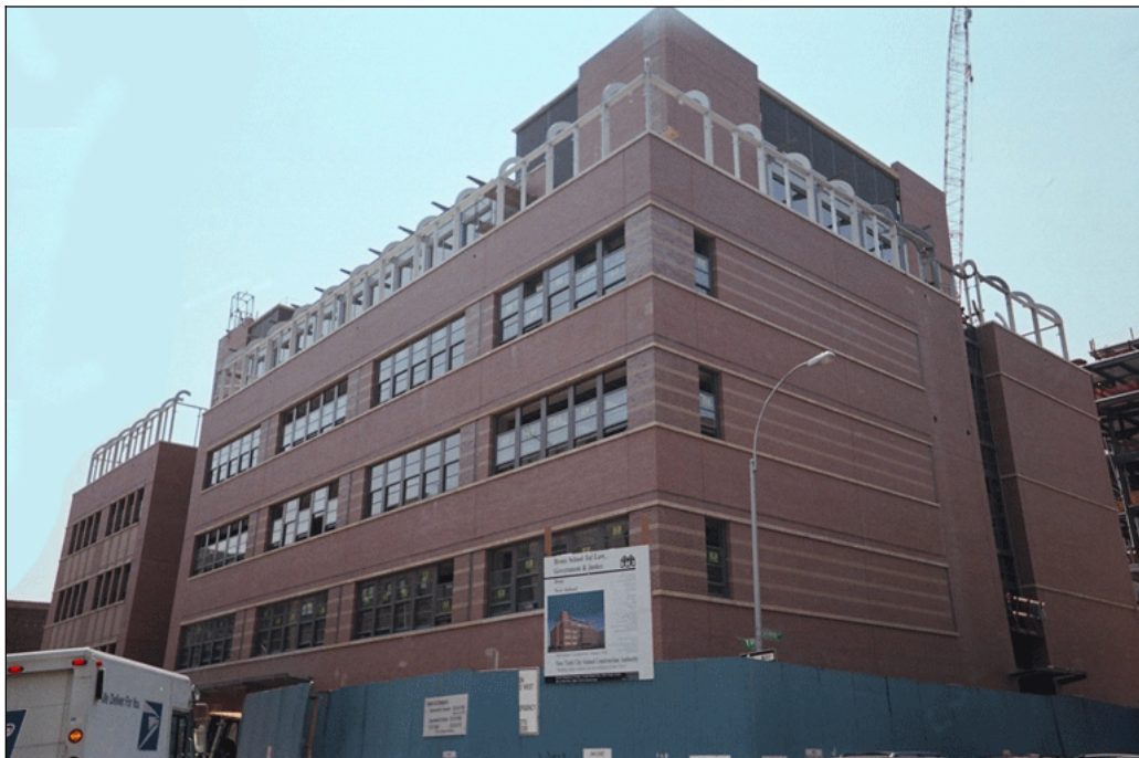
Figure 1: Construction Phase of Bronx School for Law Government & Justice
