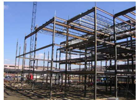
Figure 2 - Steel erection underway
