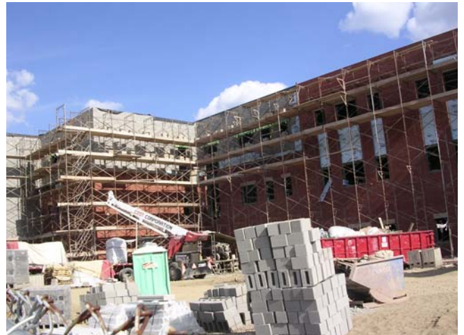
Figure 1 - Mason scaffolding around building footprint.
