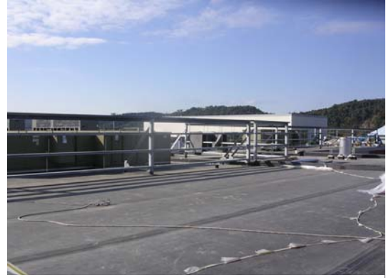
Figure 3 - EPDM Roof System on AAHS
