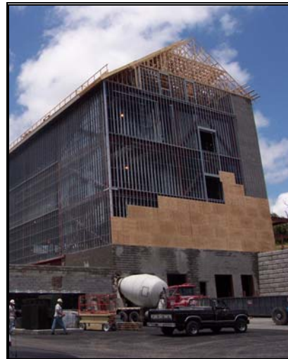
Figure 3: Light gauge steel framing with plywood sheathing 1
