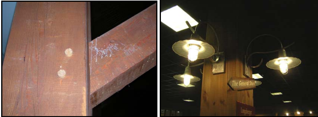
Figure 30: Examples of Steel Tube Columns Disguised as Wood in Situ 2
