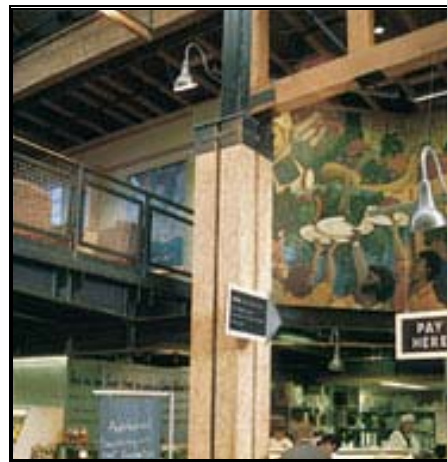
Figure 32: Engineered Wood Column Sample 4
