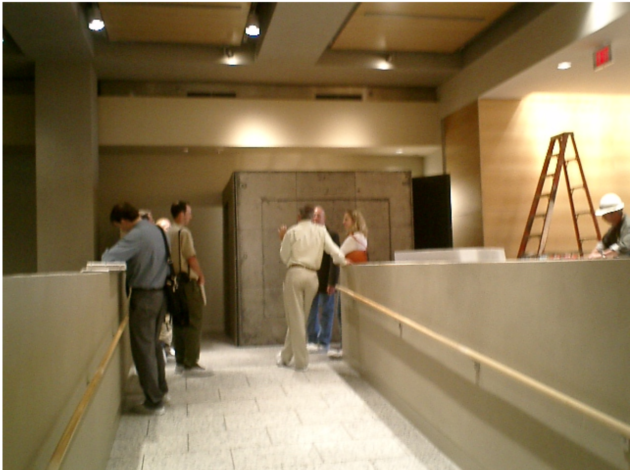
Photograph of Handicapped Stairwell During Construction
