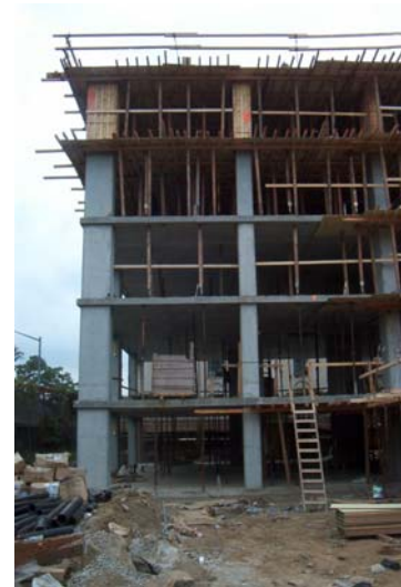
Figure 3: Concrete framing (photo courtesy GPI)
