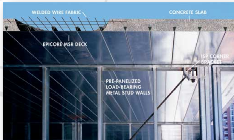
Figure 22.A: Epicore MSR Composite Floor System (www.infinitysystems.com)
