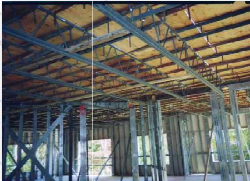
Figure 1: First Floor Hambros Joist Composite Deck System
