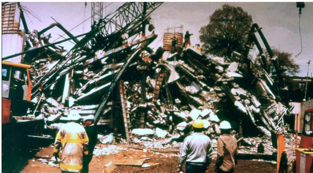
Figure C4. Debris Pile from collapse of L'Ambiance Plaza
