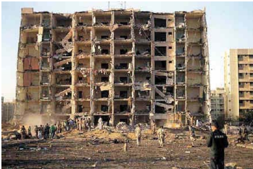
Figure C21. Side of building facing the explosion (source: http://en.wikipedia.org/wiki/Khobar_Towers_bombing )
