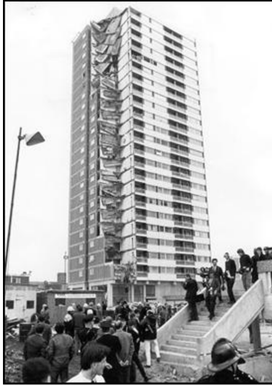
Figure C1. Ronan Point after collapse
