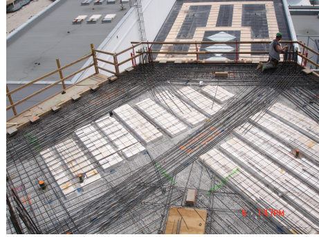
Figure 5: Filigree Construction Photo
