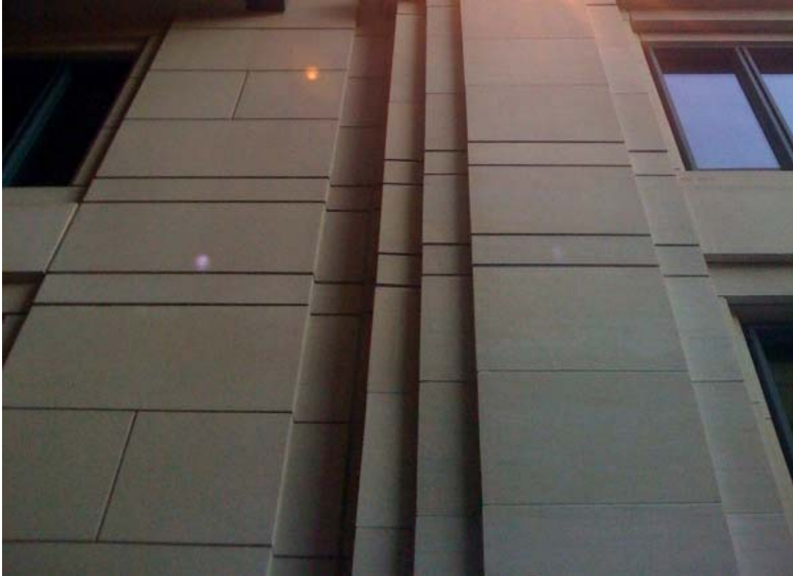
Picture 7.13-Precast (left) and Limestone (right) Side by Side
