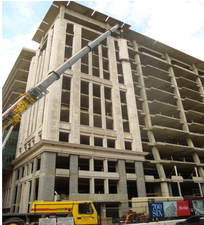
Picture 3.8-Precast Being Hung
