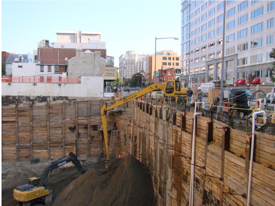
Picture 3.2-Extended Boom Excavator
