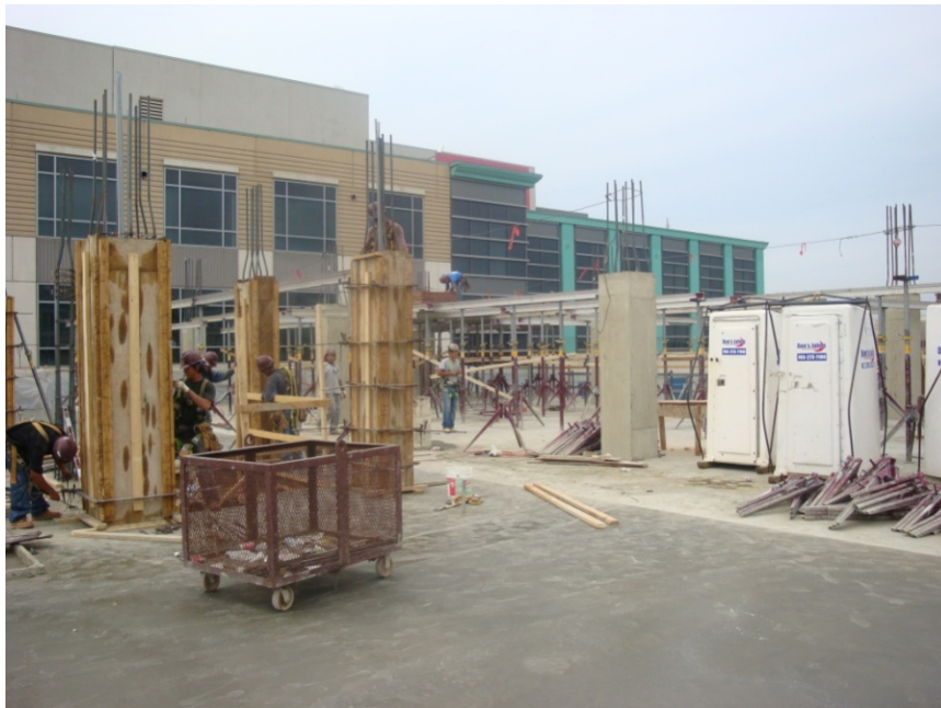
Picture 3.4-Column Formwork
