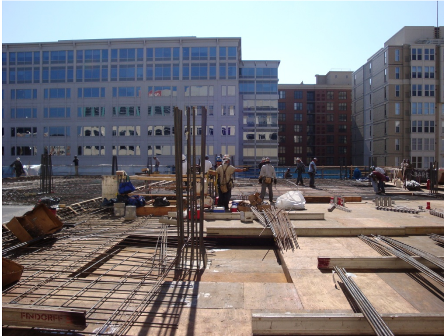
Picture 3.5-Suspended Slab Formwork
