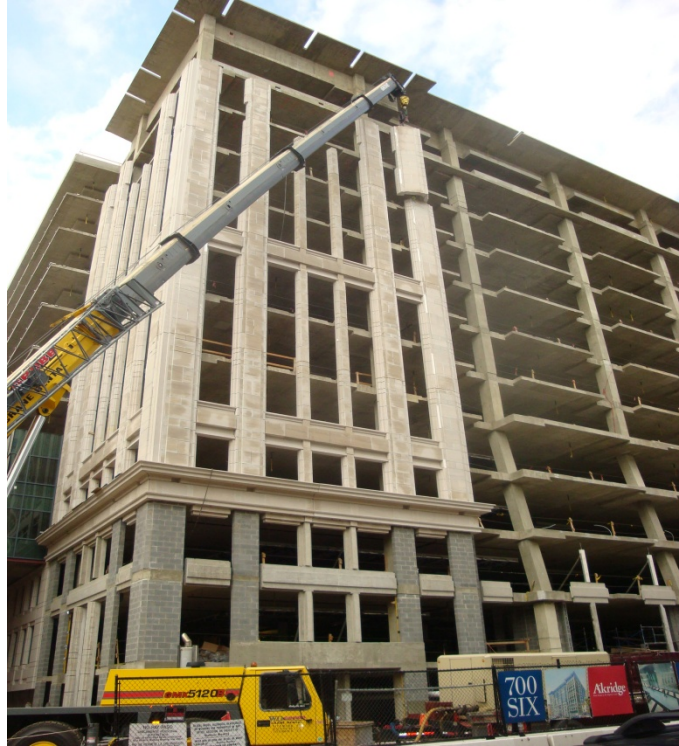
Picture 3.19-Concrete Superstructure
