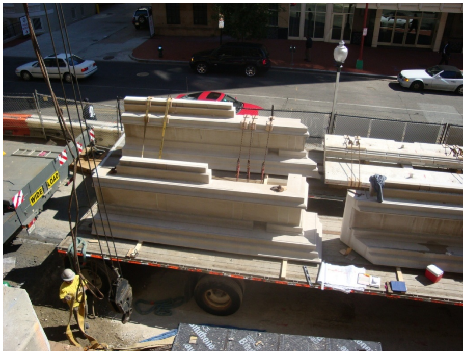
Picture 3.7-Precast Pieces
