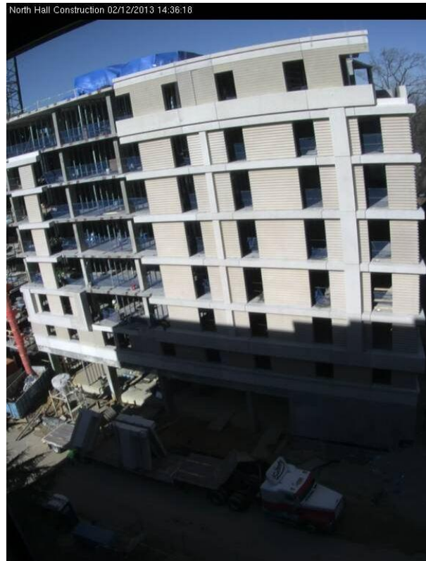
Figure 24: Precast Panel Delivery, Photo Courtesy of Grunley Construction Company
