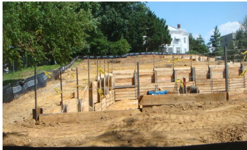
Figure 8: Material Storage/ Staging Area Photo Taken By: Brandon Tezak
