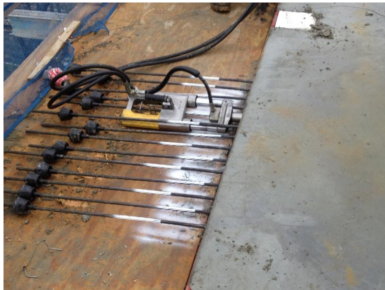
Figure 6: Post-Tensioned Tendon Stressing, Photo Taken by Brandon Tezak
