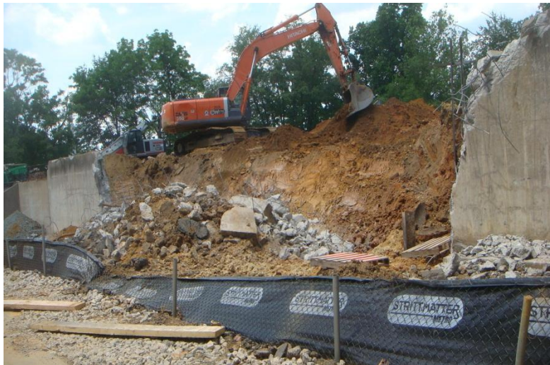
Figure 5: Large Retaining Wall Demolition Photo Taken By: Brandon Tezak
